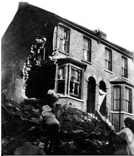
1. Church Terrace.No2.WW1 Gotha Bomb Damage
