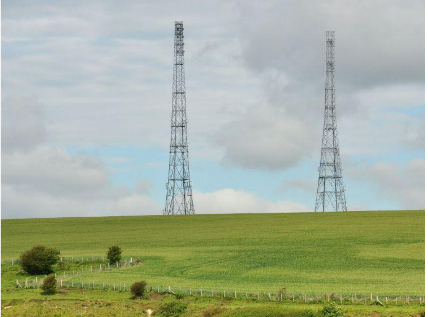
Swingate transmission towers
